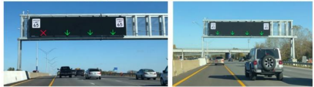
Over $5M I-670 Hard Shoulder Running (SmartLane)
